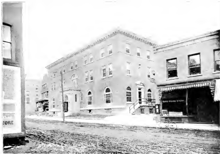
NEW Y. M. C. A. BUILDING, WINSTED
